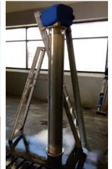
Pic 7 Cement job performed.
