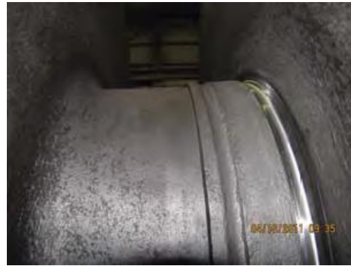
Severe shaft erosion
